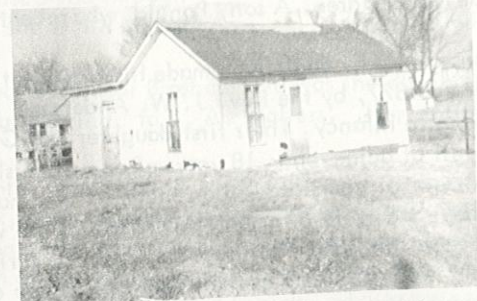
Pictured above is the three-room house built by Timothy Cusick in Brashear in 1877. Courtesy Willard Cusick
